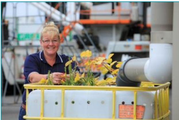
Alliance staff installing downspout stormwater treatment boxes at a marine terminal.
